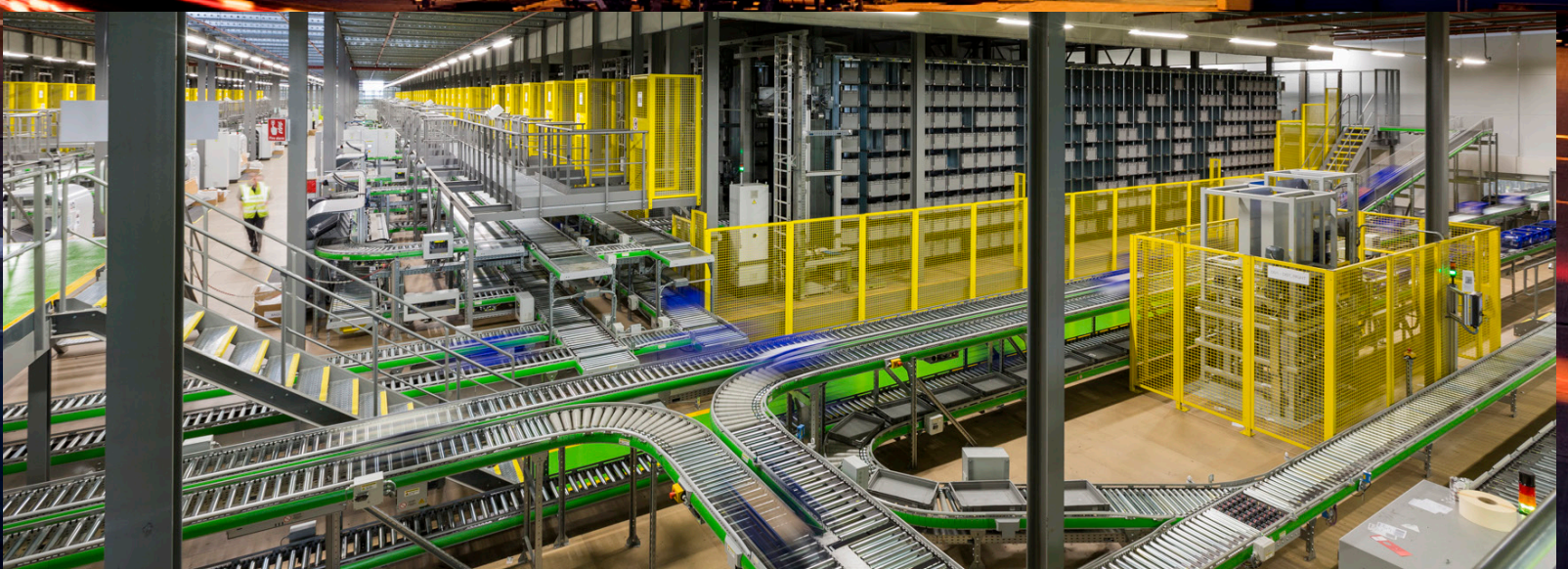
BBOX FACILITY AT CASTLE DONINGTON
