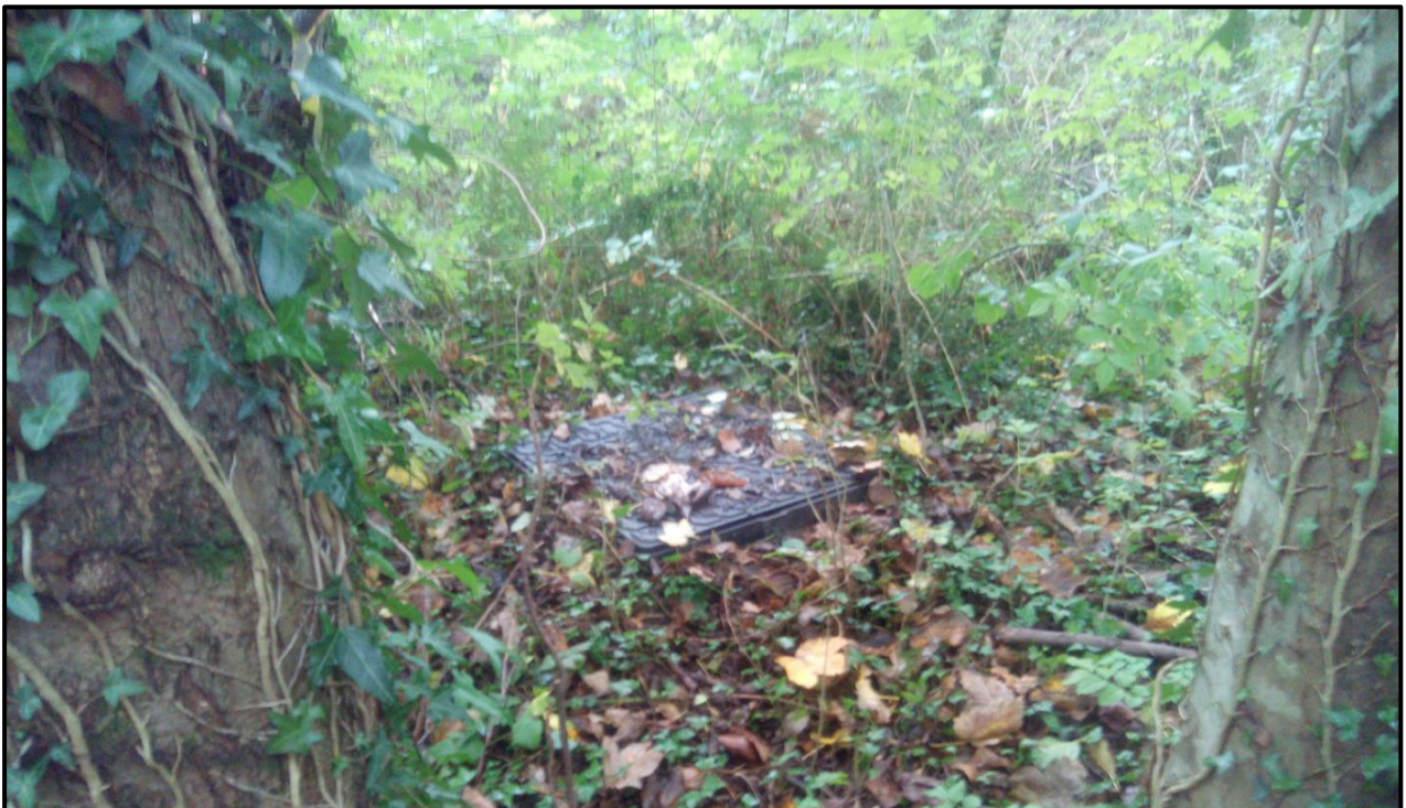
Plate 4 Observed manhole covers within wooded area
